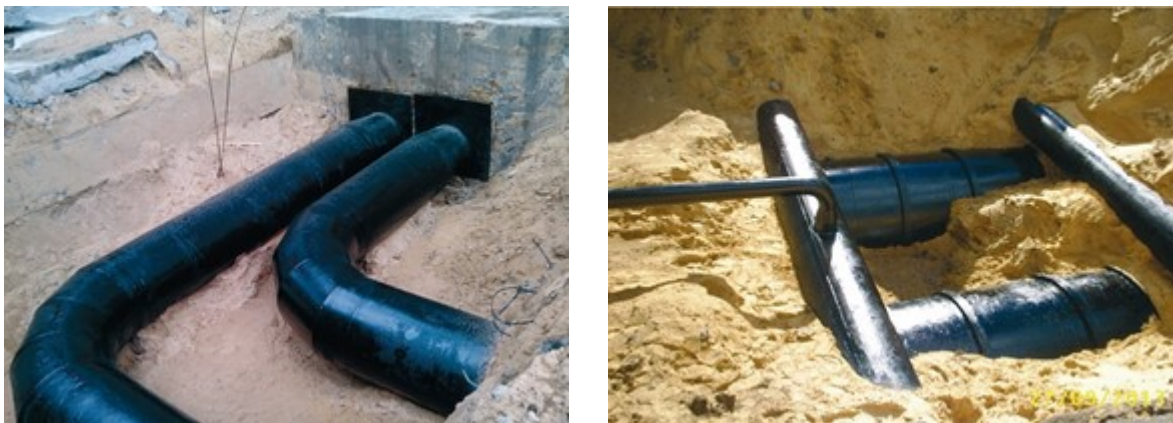
Figure 1-1: ESWS pipes (after excavation) (ref. to National Report: First Topical Peer Review Ageing Management. State Nuclear Regulatory Inspectorate of Ukraine. Kyiv 2017 www.ensreg.eu/sites/default/files/attachments/ukraine.pdf
